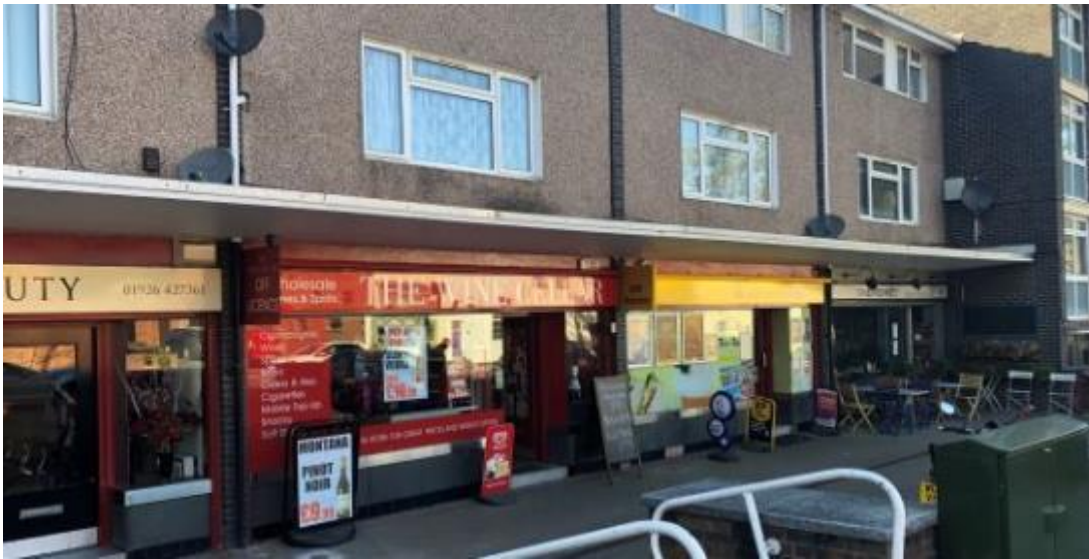
17 Binswood Street Local Shopping Centre
